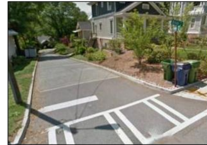
Porous Concrete - Felder St
