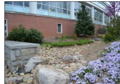
Bioswale - Klaus Building - GT campus
