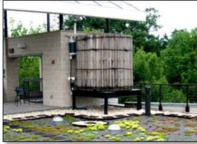
Cistern & Green Roof - Southface
