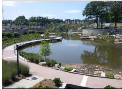
Wet pond, wetlands bench, sewer capacity relief, urban reforestation - Historic Fourth Ward
